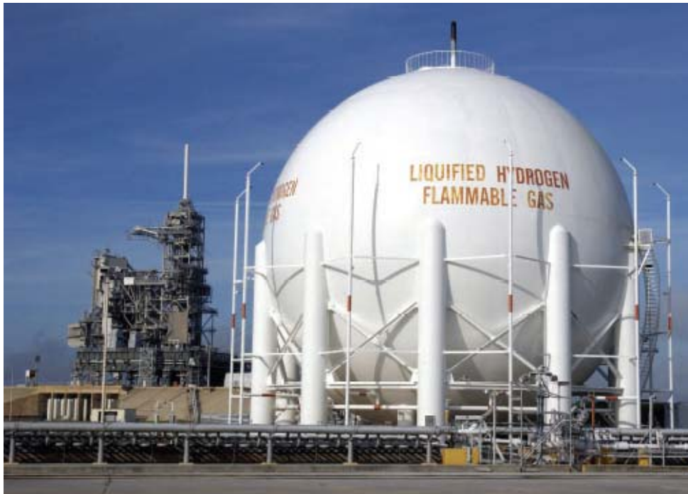
Figure 32. Complex 39 Liquid-Hydrogen Storage Facility
