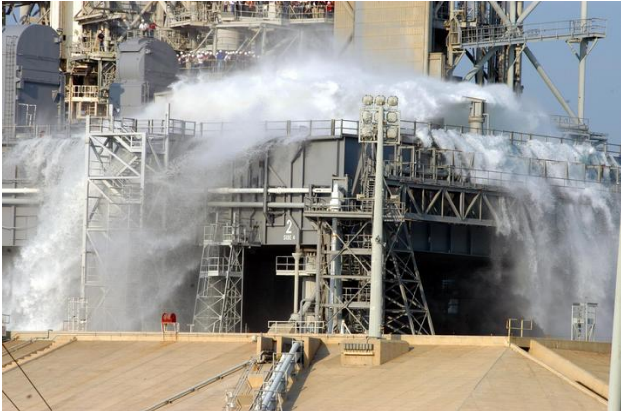
Figure 28. Launch System Undergoes an All-Up Water Deluge System Test
