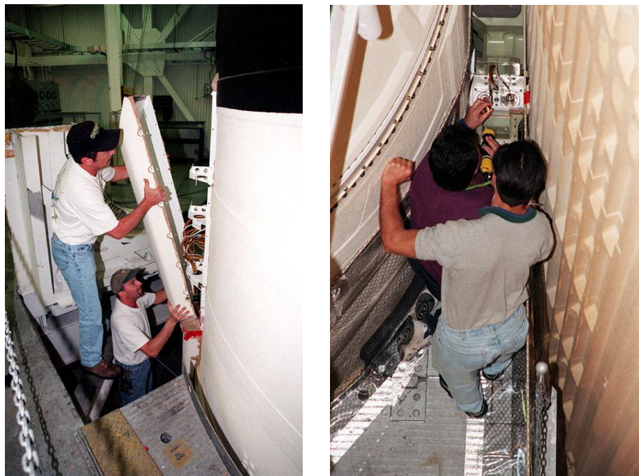
Figure 34. Example SRB Subsystem Installations and Unplanned Work
